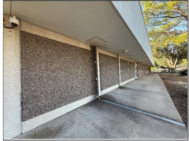
Photo #2 View of the asbestos-containing exterior rock wall panels with asbestos-containing edge wall panels
