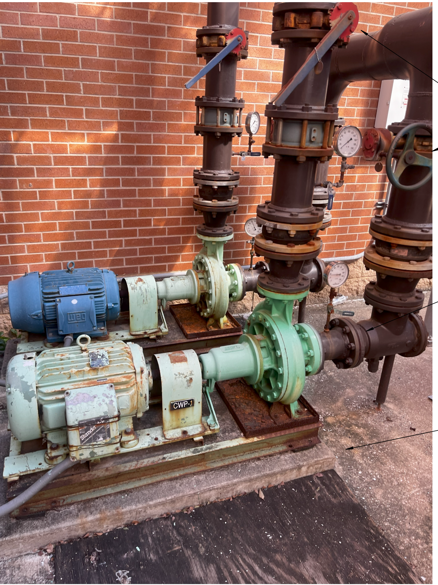
EXISTING CONDENSER WATER PUMPS
