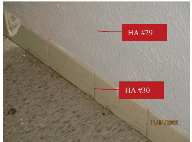
Photo 22: View of HA #29: ACBM plaster wall (crow's foot) & HA #30: ACBM ceramic cove base (tan).
