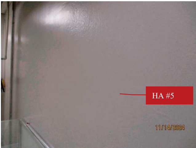
Photo 5: View of HA #5: ACBM plaster w/ texture (smooth)
