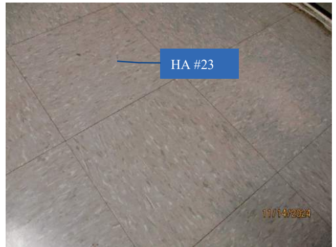
Photo 18: View of HA #23: Non-ACBM 12" x 12" (gray w/ gray & white flecks) w/ mastic.
