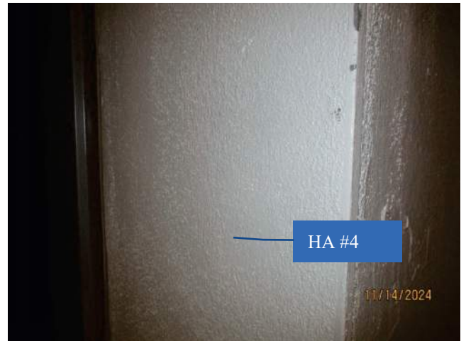
Photo 4: View of HA #4: Non-ACBM concrete wall w/ texture (sandy).
