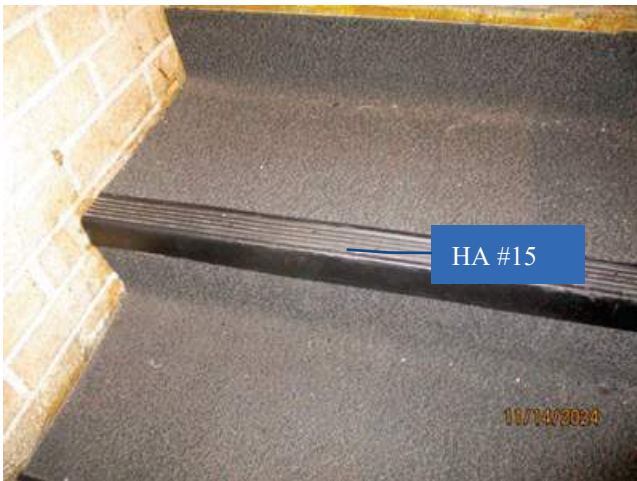
Photo 11: View of HA #15: Non-ACBM vinyl stair cap.
