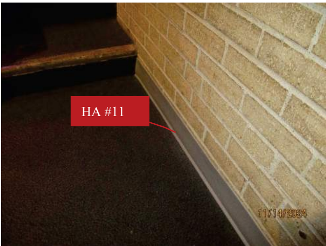
Photo 7: View of HA #11: ACBM black mastic associated with 4" cove base (gray) w/ adhesive.
