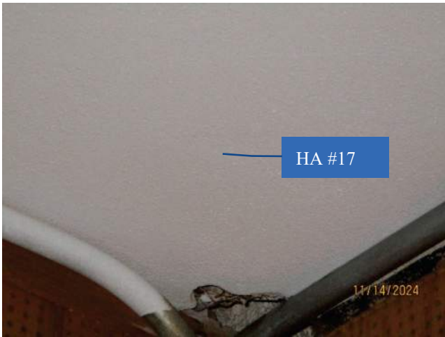
Photo 13: View of HA #17: Non-ACBM plaster ceiling (sandy).
