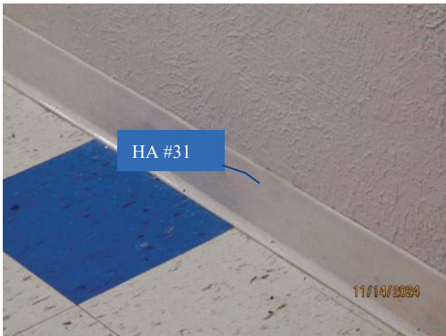
Photo 23: View of HA #31: Non-ACBM 4" vinyl cove base (white) w/ adhesive.
